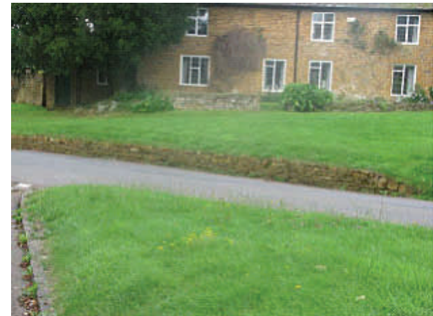
The low retaining wall outside Oriel House
