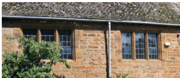
Village Hall - Stone mullioned windows with metal casements
