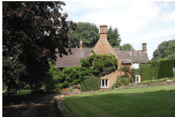
Tanners Pool: a modern re-build of an older property
