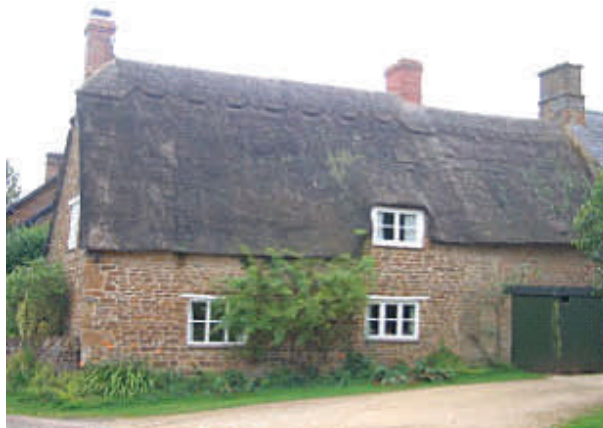
Thimblestone Cottage - Ironstone rubble with one of the few remaining thatches
