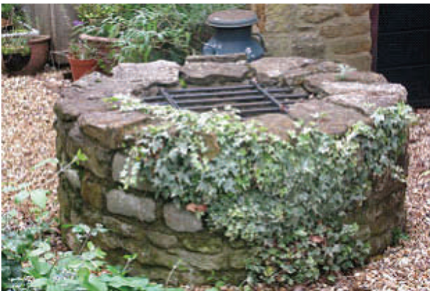
The well at Dairy Well
