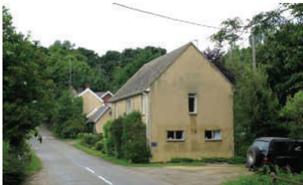
Tanner's Cottage — under the concrete render lies a Victorian red brick structure:
