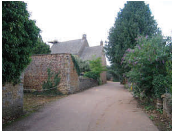
Kenhill Road leading to the scheduled monument
