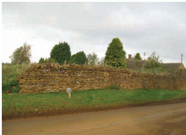
Partially demolished stone wall along Rattlecombe Road
