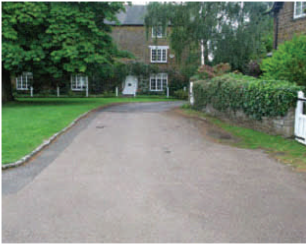
Outside Mulberry Cottage, the rather pristine green contrasts with the soft verge now slightly eroded by parking.
