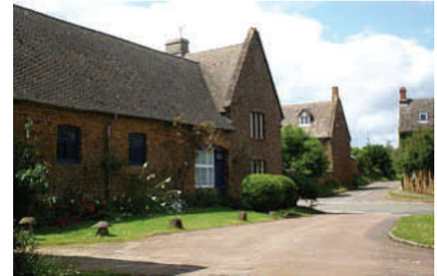
Longworth, formerly one of the village shops
