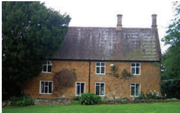
Above: Oriel House - the steep pitch of the ties roof suggests it was once thatched
