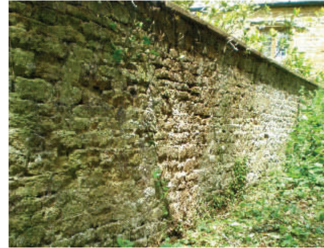
Striking boundary wall
