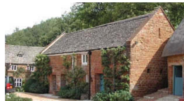
Outbuildings of Barn House
