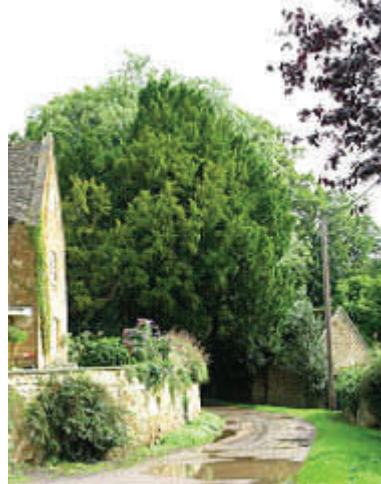
Manor Farmhouse: retaining wall and vegetation
