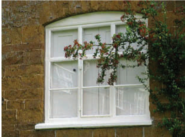
Manor Farmhouse window with internal shutters
