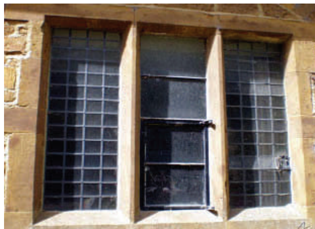
Traditional stone mullioned window
